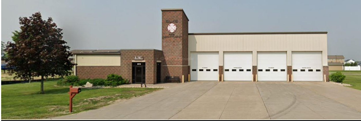
Figure 16: Fire Station 2 - 2010 10th St, Silvis IL 61282
